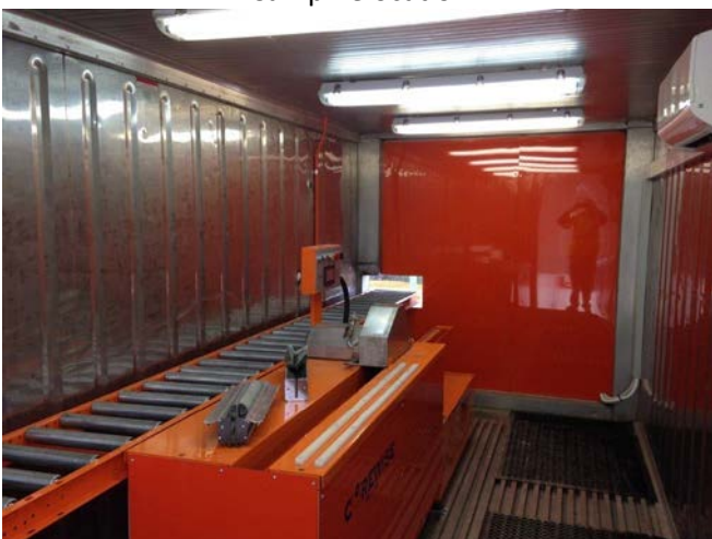
Core Saw Installation
